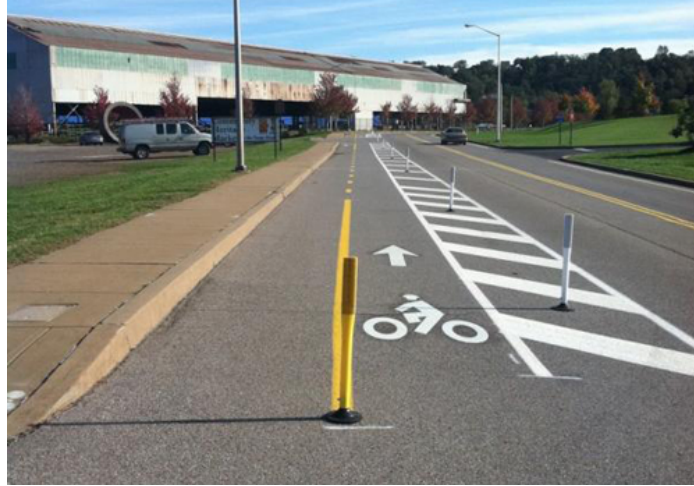
Two-way bicycle lane in Munhall
