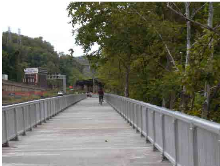
Millvale Trail Connection, elevated trail section to replace section of trail along the North Shore of the Allegheny River, between the 31 st and 40 th Street bridges.
