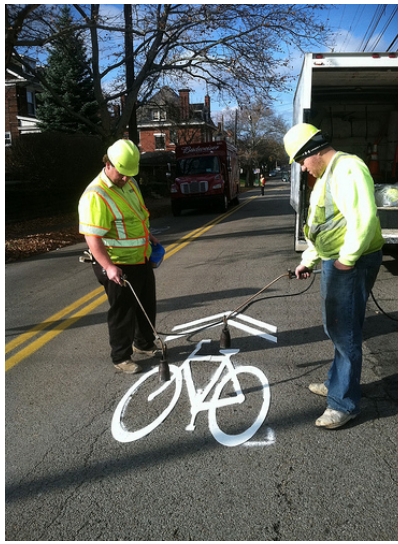
Workers install sharrows on Friendship Ave and Millvale Avenues in Bloomfield
